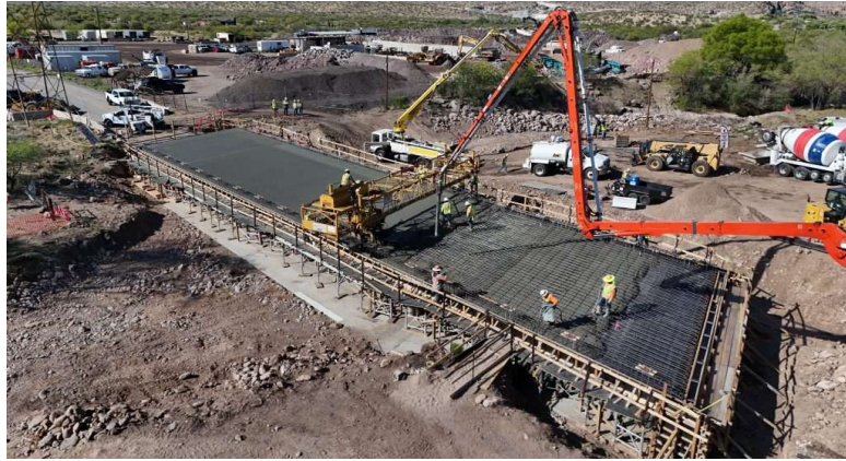
Photo 2– Panther Drive Bridge is Under Construction to Address Flooding Concerns
