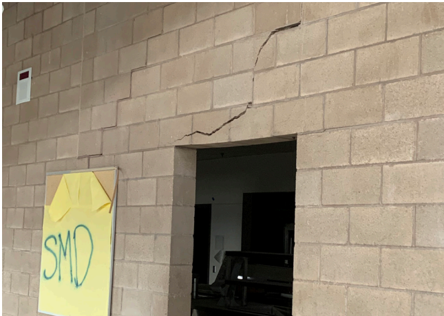
Cracks in walls
