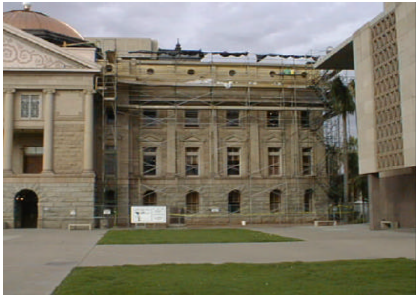
Photo 1 — Construction at the Capitol Building
