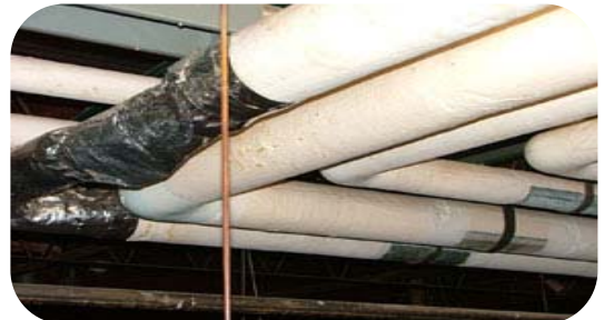
Photo 8: Repaired water lines at UA's Centennial Hall
