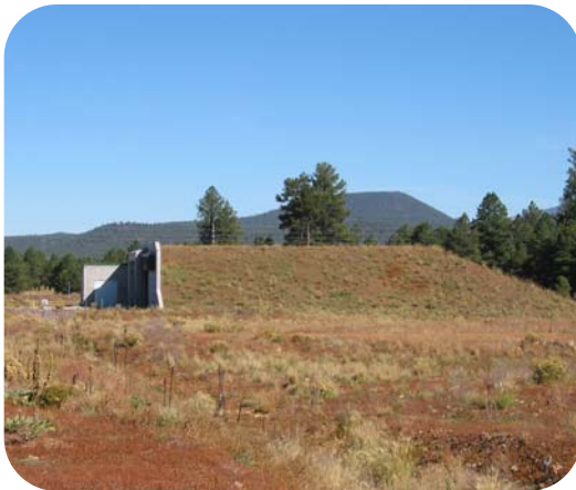
A concrete "igloo" used to store items such as rocket motors.
