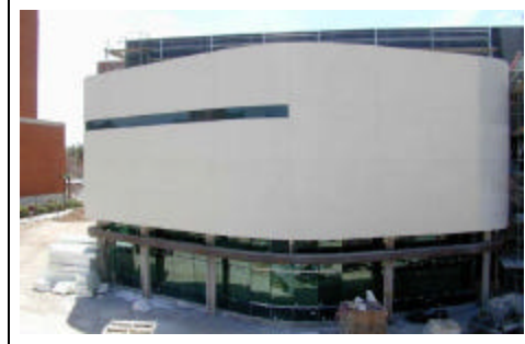
Photo 4: University of Arizona Student Memorial Union Kiva Under Construction
