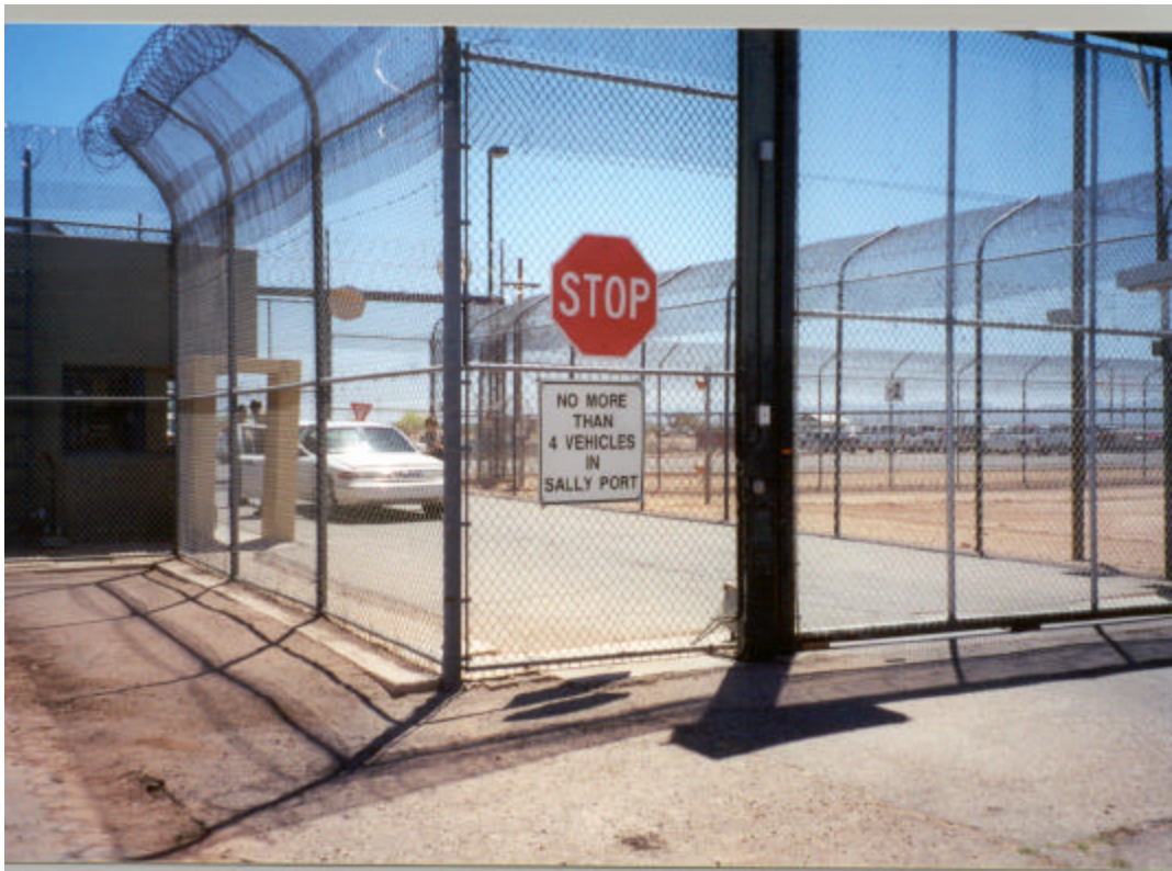
Photograph 15 Complex vehicle entrance at ASPC-Tucson
