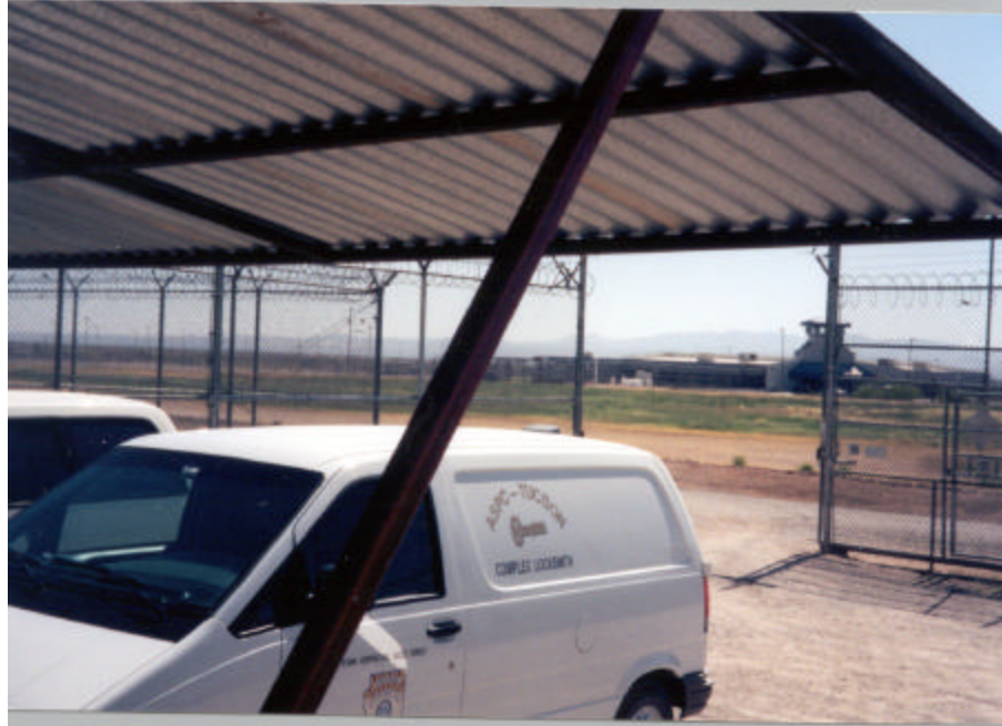
Photograph 9 Open gate to lock shop area at ASPC-Tucson
