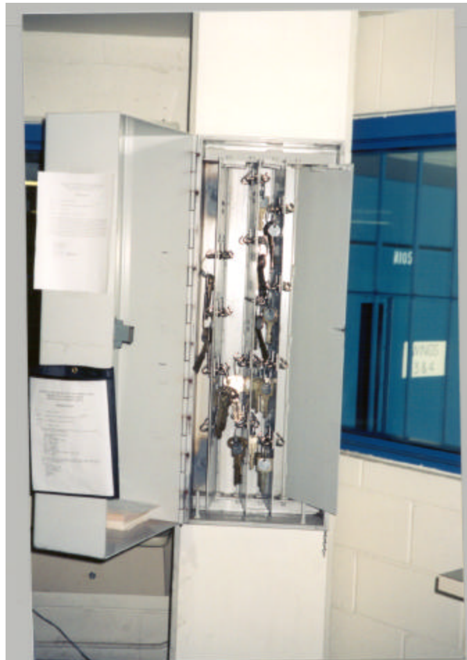
Photograph 6 Secured keys in Northwest Control Room at ASPC-Eyman
