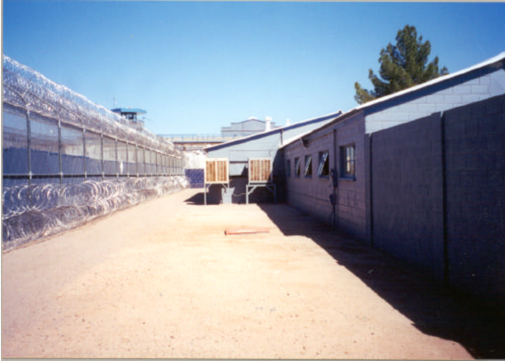
Photograph 13 Blind area near Lincoln Dormitory in East Unit at ASPC-Florence
